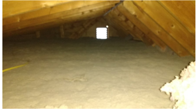
Additional cellulose added to attic.
