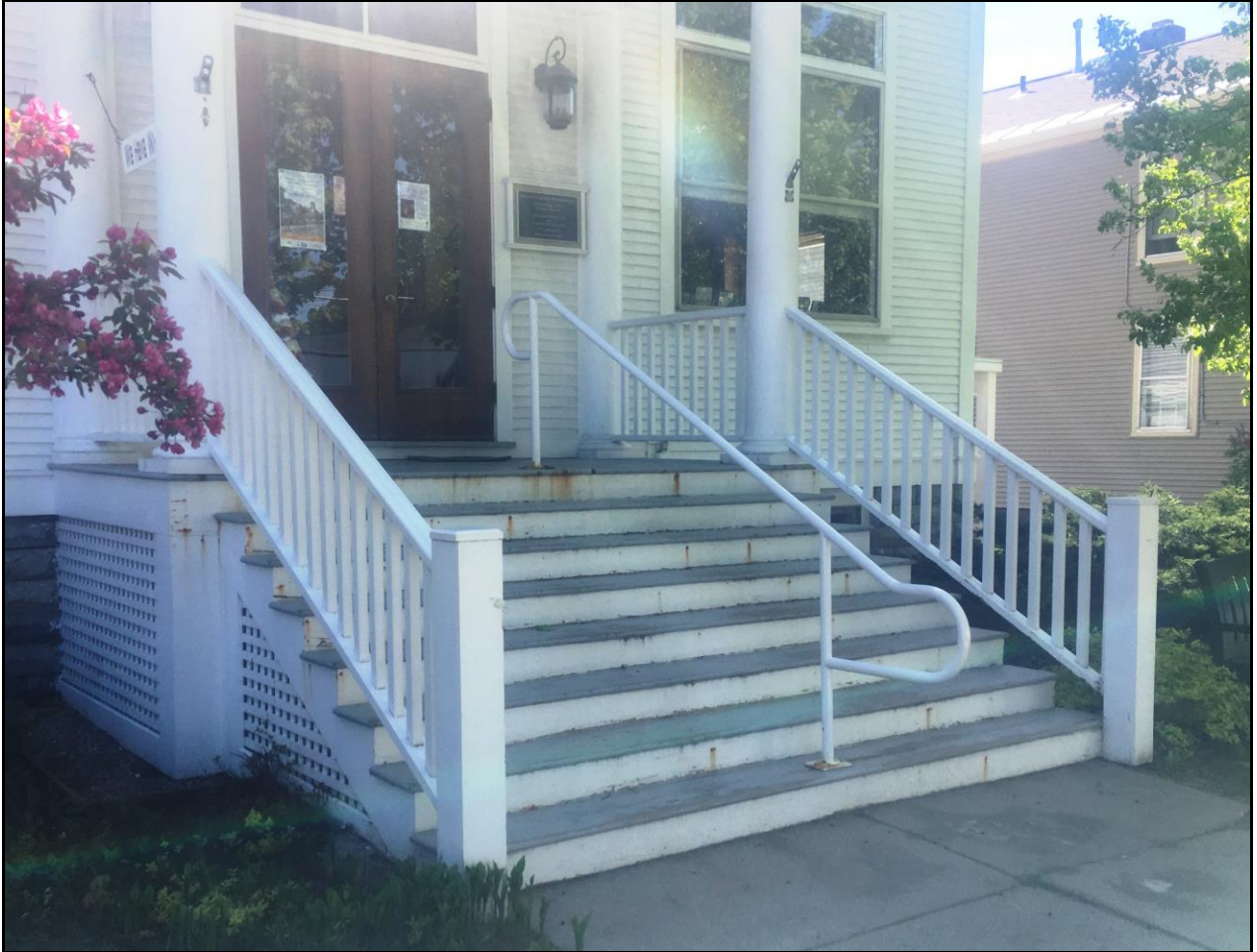
Figure 1. Lawrence Lane view of the stairs.
