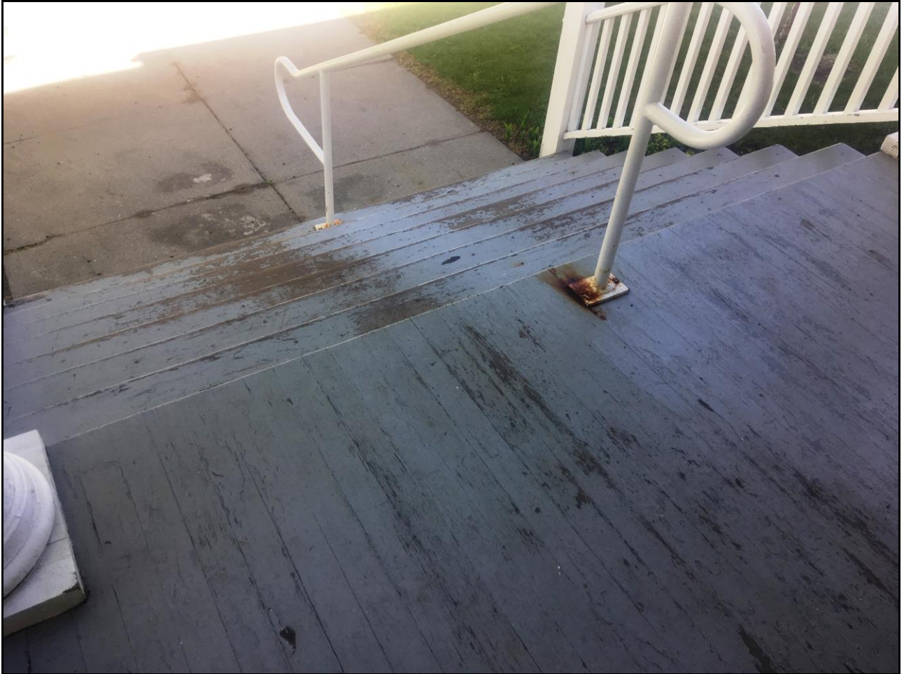
Figure 3. Deck view of Library stairs.
